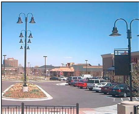
Figure 9.3-37 Example of appropriate light fixtures
